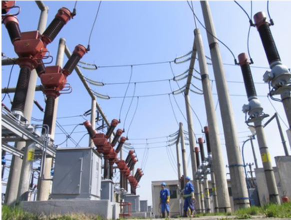
Biogas Plant: Filipestii de Padure, Prahova County
