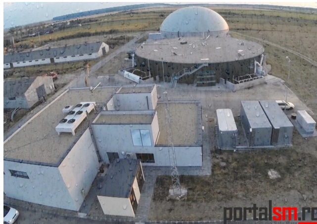
Biogaz plant: Ardud City, Satu Mare County
